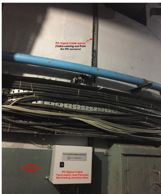
Fig. 4: PD Signal Layout & Termination Box Mounted
