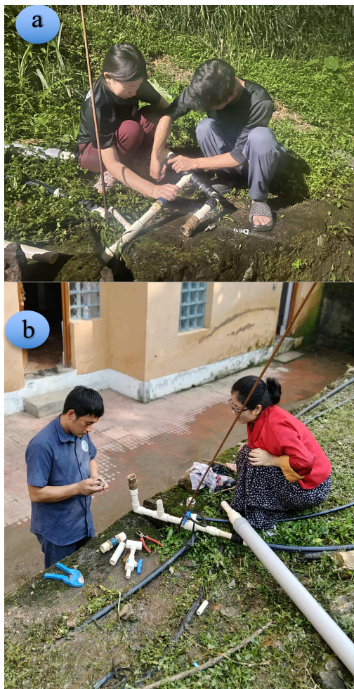
Fig. 8: Development of the working model: (a) fixing the pump fittings and checking alignment; (b) sealing potential leakage points at the pipe joints
