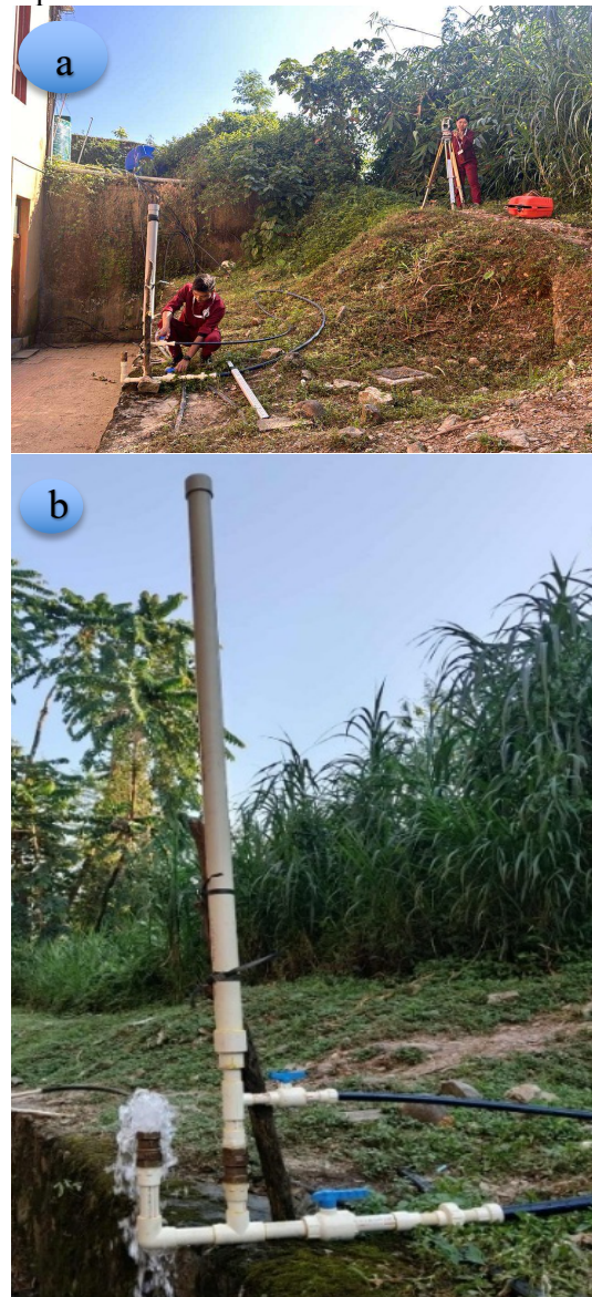
Fig. 9: Field testing: (a) installation of the hydraulic ram pump at the prepared site; (b) the pump in operation, delivering water to the elevated outlet
