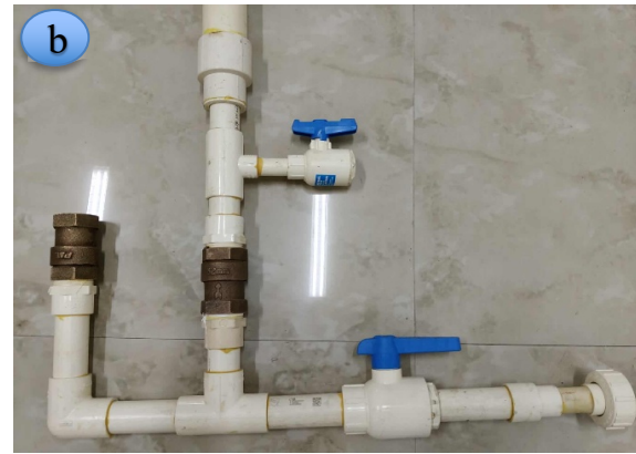
Fig. 6: Locally procured parts used to build the prototype: (a) individual components of the hydraulic ram pump before assembly; (b) the same components after assembly into the pump body
